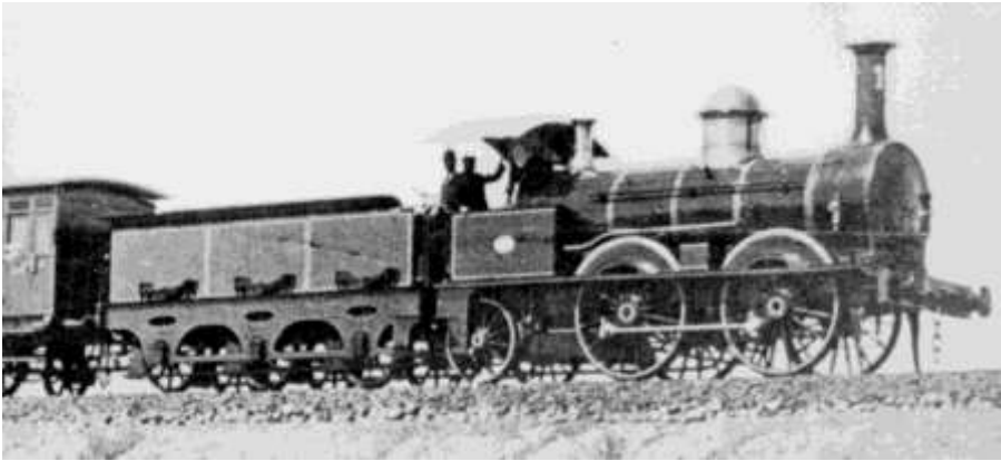
Figure 1 – Engine No 1 on the way to Parramatta, shortly after the official opening, displaying a useful Australian modification – a corrugated iron cab roof, 1855
